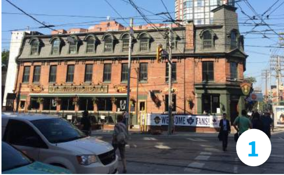
667 King Street West: listed
