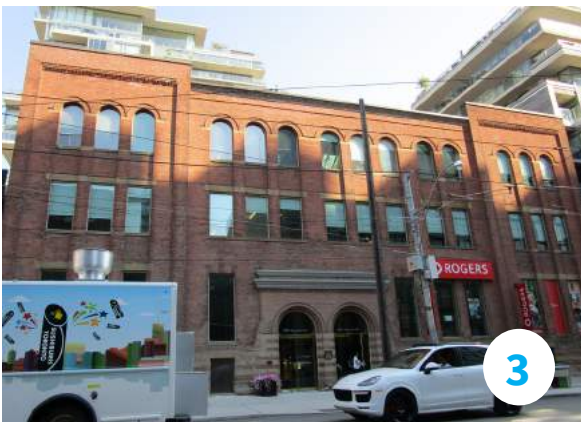
662 King Street West: listed
