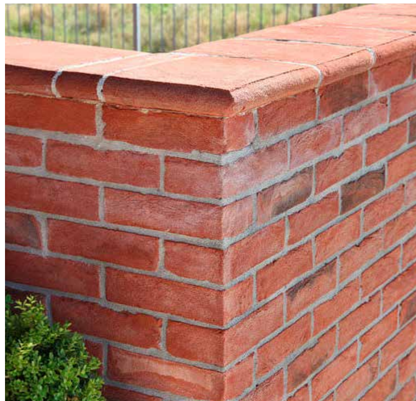
WALL DETAIL CLAY BRICK WALL COPING
