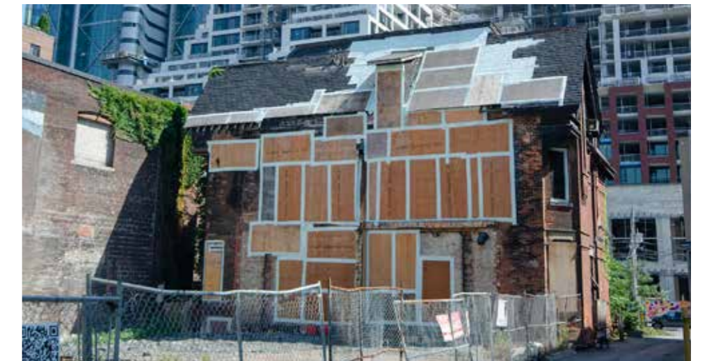
Existing rear condition
