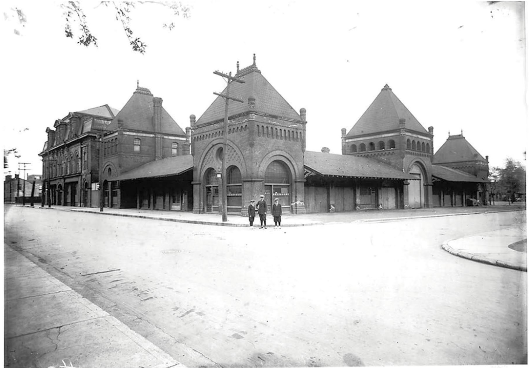
Old St Andrews Market, Richmond St W 1971
